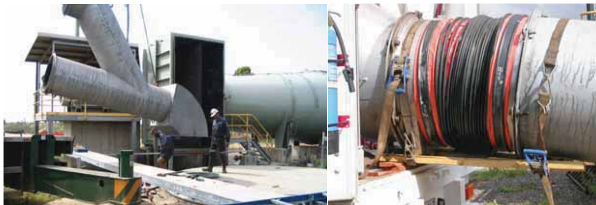
Figure 4.4 Positioned shaft cap, injection elbow and flexible elbow to GAG and aligning GAG flexible connection.
