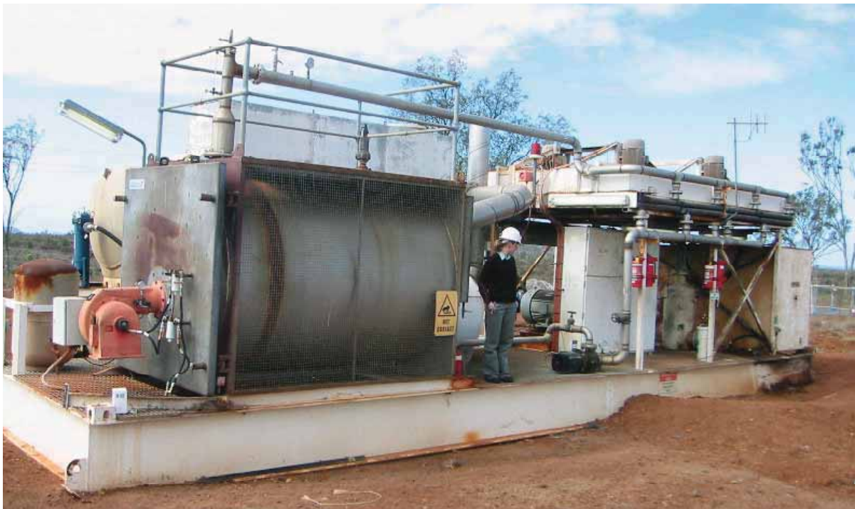
Figure 2.2 Tomlinson unit on mine site
